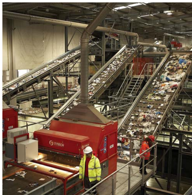
The waste industry says that modern materials recovery facilities can provide high quality recyclable resources. The photograph is of the materials recovery facility operated by Biffa Waste Services at Trafford Park, Manchester that processes plastics, aluminium, steel, paper and card.
